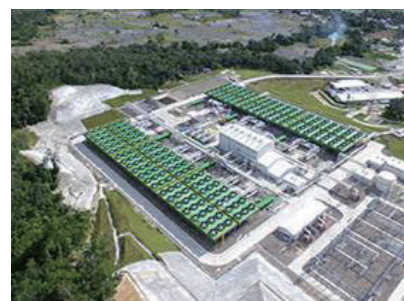
Total commissioning for Sarulla Geothermal Power Plant in Indonesia
