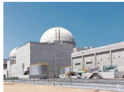
I&C commissioning S1, S2 for Baraka Nuclear Power Plant in the UAE
