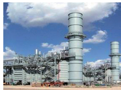
I&C commissioning for Thermal Power Plant in Saudi Arabia
