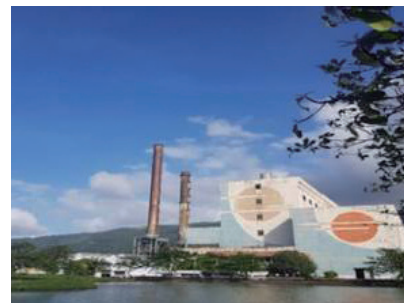
O&M for Malaya Thermal Power Plant in the Philippines
