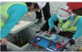
Earthing Resistance Test (330kV SWYD)
