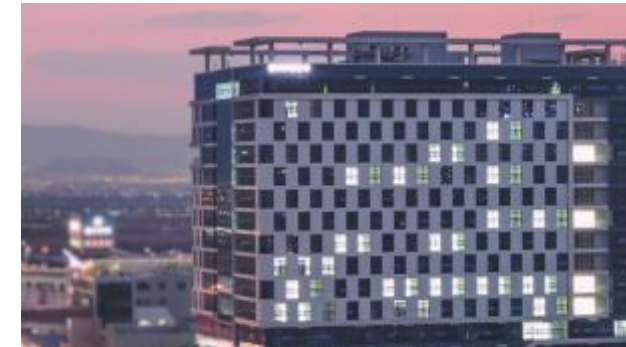
BUSAN VENTURE TOWER (Head Office)
