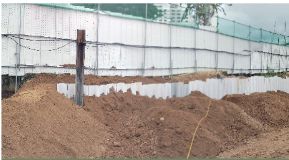
Uijeongbu Soil Remediation Site, Korea
