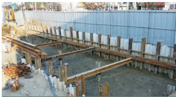
SK Deuk-ryang Gas Station, Korea
