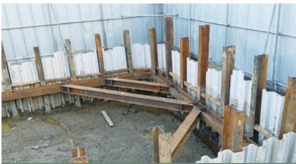
SK Deuk-ryang Gas Station, Korea
