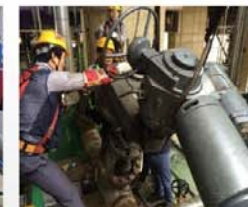
The VALVE MEDIC TEAM (valve maintenance organization) is repairing the MOTOR OPERATED VALVE.
