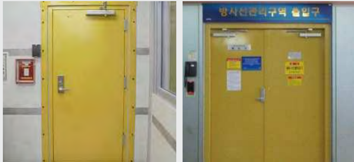
Hanbit Unit 5 & 6 Access Control Building
