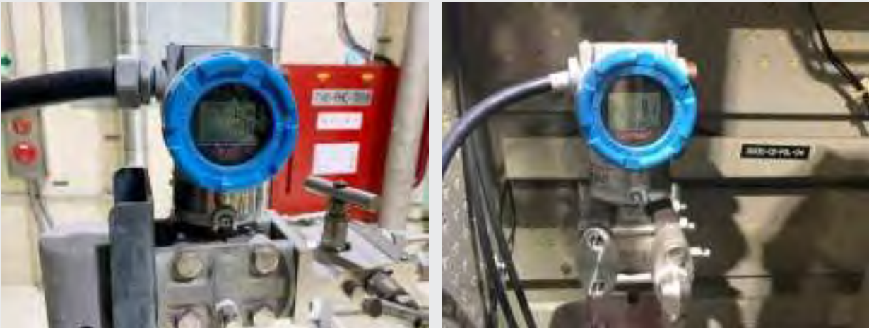
Wolsong Unit 1 & 2 Turbine Building
