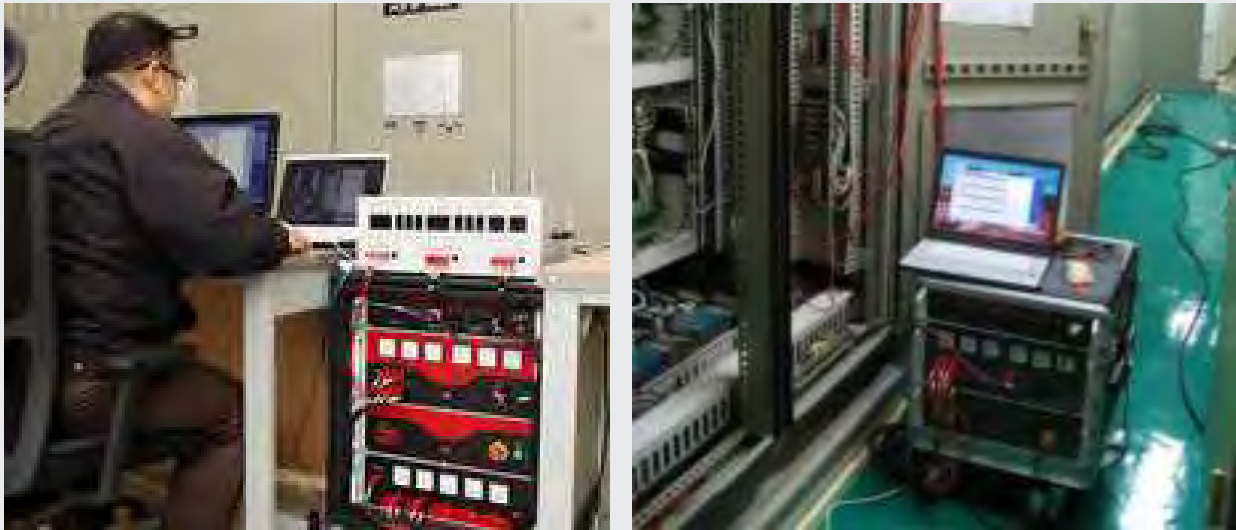
Conducting Comprehensive Test
