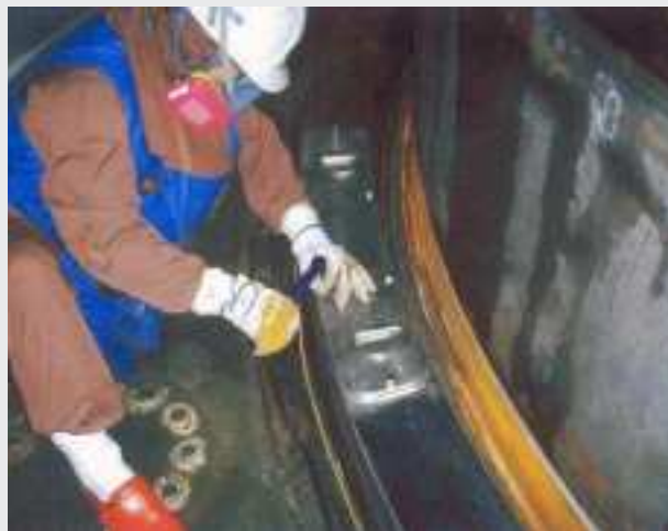
Vent Cover Installed
