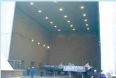
Shot & Painting Facility
