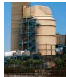
Experience : 890 MW TECO Big Bend Station, Units 1 & 2 Location : Apollo Beach, Florida, USA Customer : TECO Start-Up Year : 1999 Capacity : 890 MWe Flue Gas Flow : 3,102,000 Nm 3 /h
