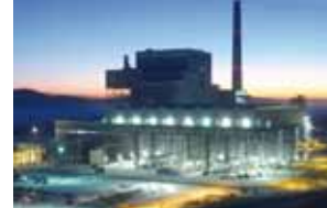
Largest CFB Scrubber is at Dry Fork Station Location : Gillette, Wyoming, USA Customer : Basin Electric Power Cooperative Start-Up Year : June 26, 2011 Capacity : 420 MWe Flue Gas Flow : 1,580,000 Nm 3 /h per unit
