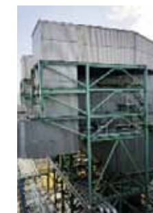
Non-Leakage GGH Cooler Design : 2 x Vertical Flow Spiral Fin-Tube
