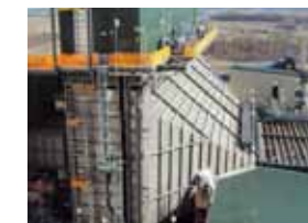
Largest Wet ESPs References in World Design : 2 x Plate Horizontal Flow Capacity : 2 x 800 MW
