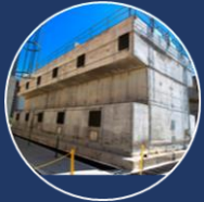
Dry storage facility for spent fuel (DICA)
