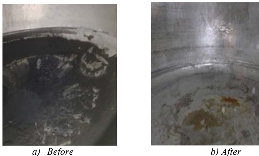
FIG. 12. Cleaning of waste holdup tanks to remove solid precipitates. (Courtesy of Pacific Gas & Electric Company, USA).
