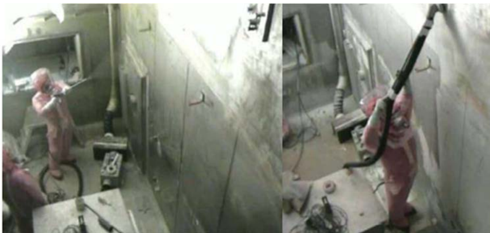
FIG. 19. Spraying of a self-drying gel onto a contaminated area and the removal of cracked gel after drying (reproduced from Ref [56] with permission courtesy of CEA, France).
