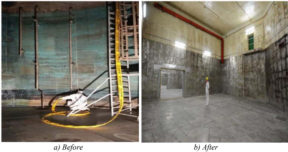
FIG. 15. Decontamination of tanks at Bohunice V1 NPP during decommissioning. (Courtesy of JAVIS, Slovakia).
