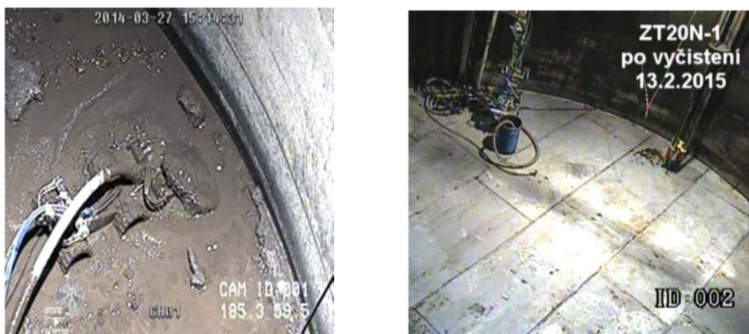
FIG. I-1. Removing of solids (cleaning) the inside of spent liquid storage tanks. (Courtesy of JAVIS, Slovakia).
