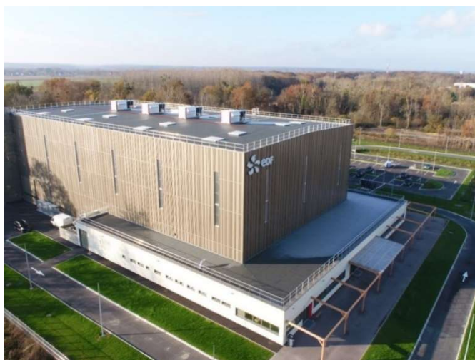
FIG. III-1. Industrial demonstrator. (Courtesy of EDF, France).
