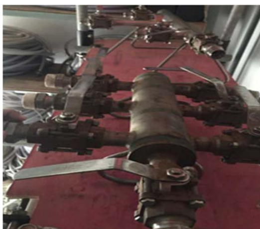
FIG. 7. Reuse of water from RCA drains during outages to minimize waste at the Angra 2 NPP. (Courtesy of Eletrobras Eletro Nuclear, Brazil).
