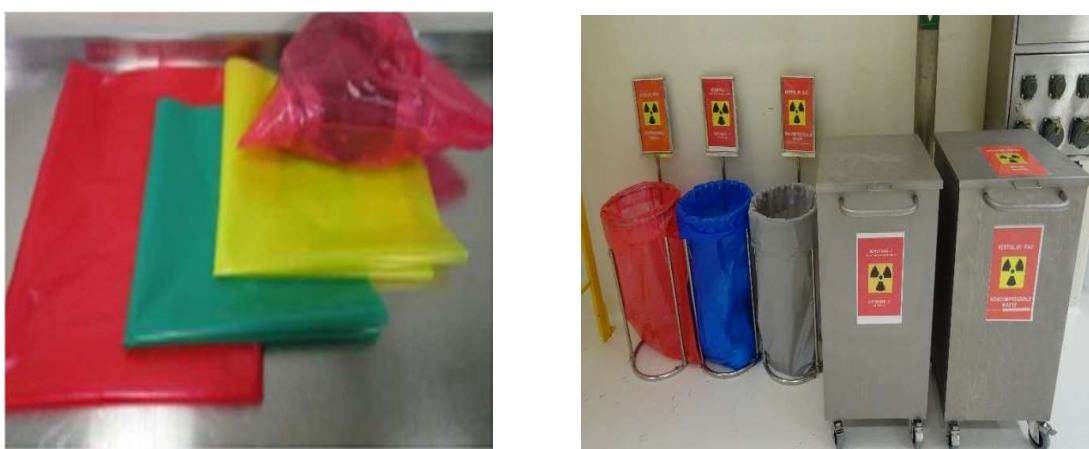
FIG. III–8. Segregation of RAW at Krško NPP. (Courtesy of Nuclear Safety Administration, Slovenia).
