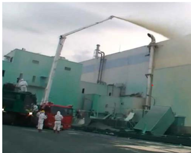
FIG. 16. Application of gel to remove contamination at Fukushima Daiichi NPP (reproduced from Ref [48] with permission courtesy of Tokyo Electric Power Company (TEPCO)).
