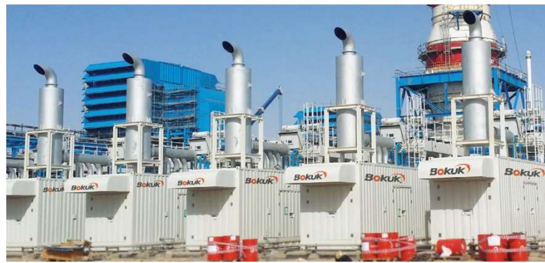
Algeria/6 x 2.5MVA Diesel Generator - 6.6kV, 50Hz, 1500rpm - with containerized enclosure
