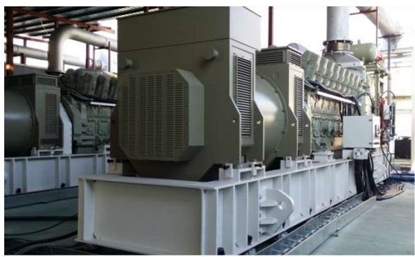
Japan/2 x 2MVA Diesel Generator - 6.6kV, 50Hz, 1500rpm - with containerized enclosure
